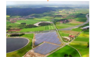
Muehlhausen, Germany , 6 MW
