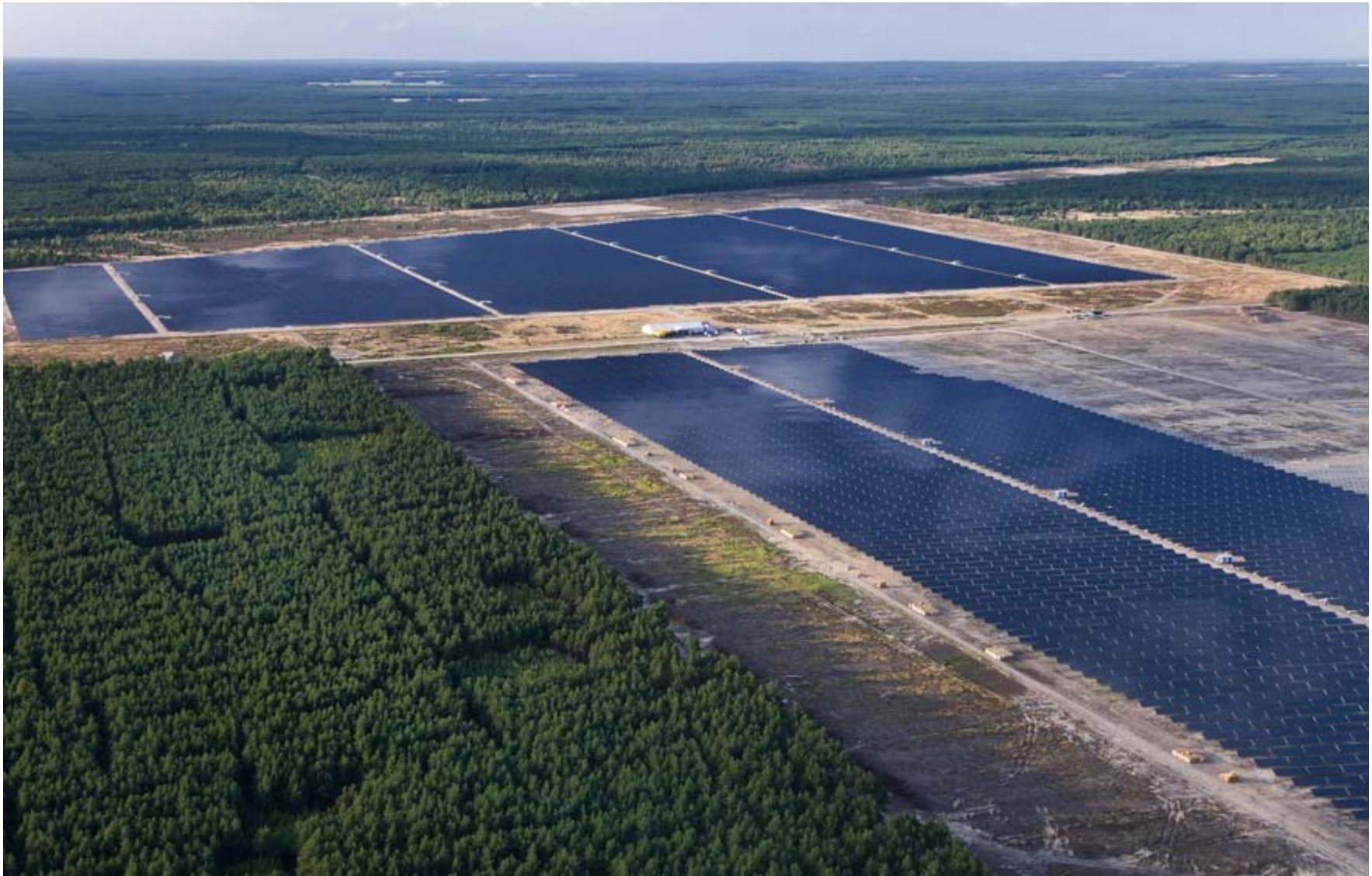
Solarpark Lieberose (Germany) - 53 MW (photo courtesy Juwi)
